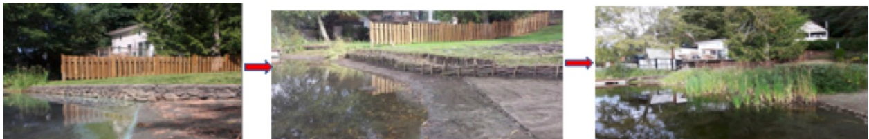
Figure 1. A stone wall (left) was replaced initially by a wattle wall and bulrushes (middle) and after a few years a more natural shoreline is in place (right).
