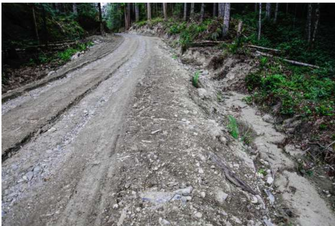
Figure 67: The two erosion channels running down the surface of this haul road and the ditch on the side of the road demonstrate how water is intercepted from its dispersed pattern in the forest and concentrated by roads, including skid roads and log landing areas. The road in this photo needs to be restored by re-routing water that is eroding the road, providing for cross drains that reduce water concentration, eliminating point sources of water siltation, and re-establishing permeable surfaces wherever possible. Reducing the area of roads throughout the watershed is vital to restoring water quality, quantity, and timing of flow; and overall biological diversity.
